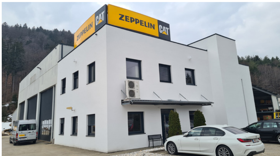
Modernized site in Villach (Austria)
