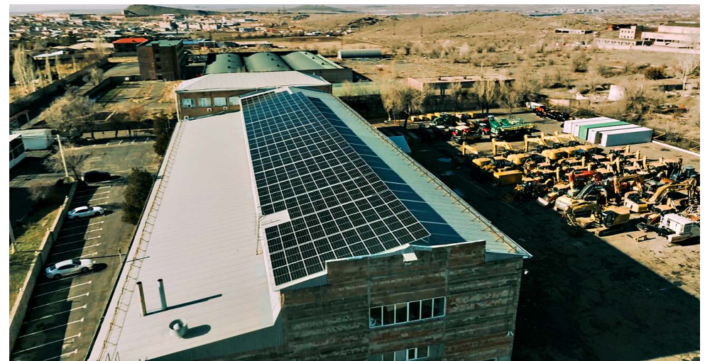
229,000 kWh of green electricity: Generated by the PV system at the Zeppelin Armenia site, newly installed in 2023
