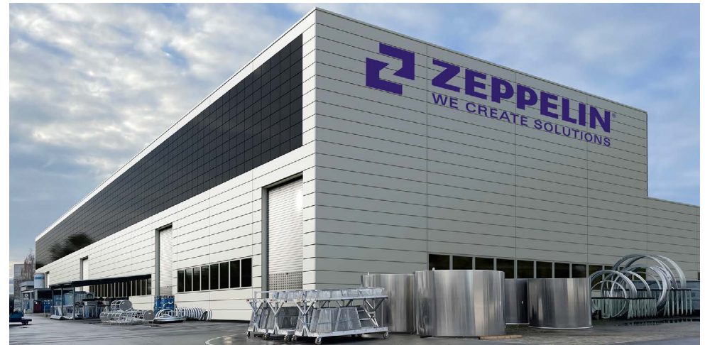
Modernization of the Ludwig-Dürr Hall in Friedrichshafen began in 2023
